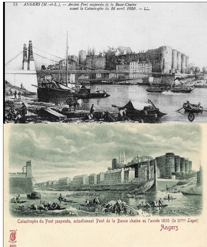
Figure 5: Angers bridge collapse.
